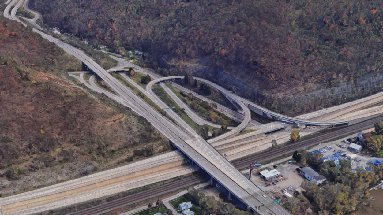
Interstate 79, PA Route 65 and Kilbuck St Interchange
